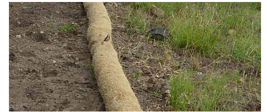
Erosion Control Log
