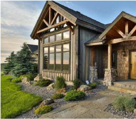
Sandstone pavers, river rock, timbers and evergreen trees are all important Colorado materials
