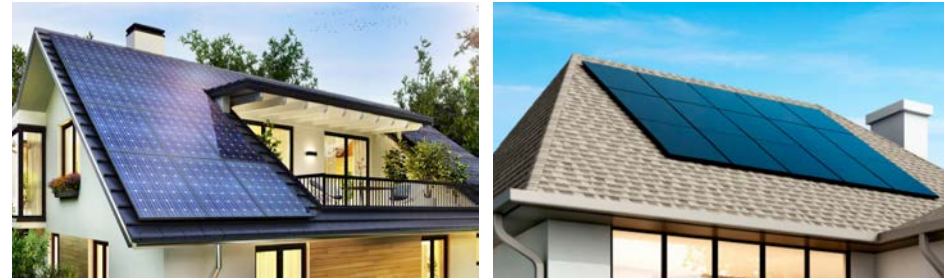
Low profile solar panels on roofs
