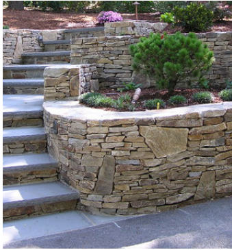
Terraced stone wall with landscape area between walls help to break up visual impact of wall
