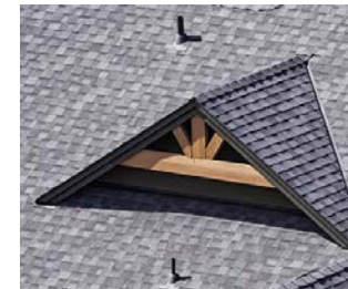
Asphalt Shingle (must have shadow line)
